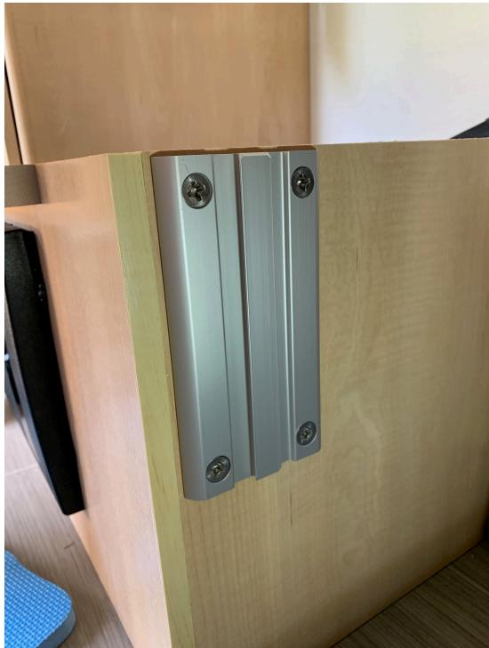
We chose to disregard the holes in provided support board and drill our own to install the mounting plate where we wanted. We put it close to the front of the seat box and almost flush with the top.
